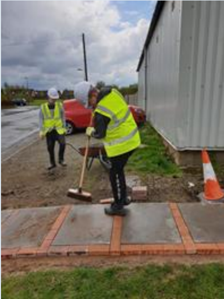
Completed disabled access at Stoneyburn Junior Football Grounds
